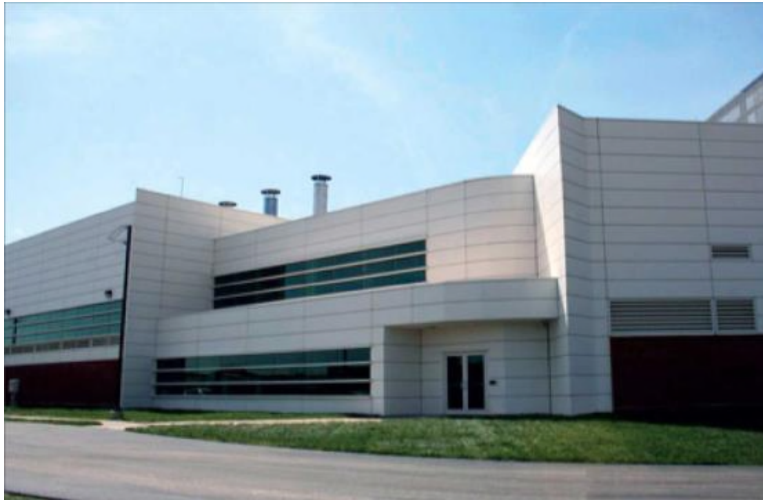
Central Utility Plant – Phase 1, Fort Detrick, Maryland
