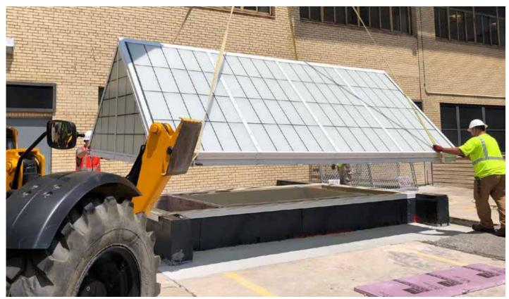
To solve a permanent equipment access problem, an opening was cut into the existing parking lot and a removable Kalwall skylight was installed.
