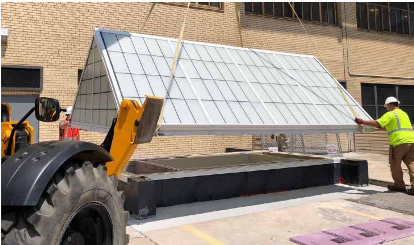
To solve a permanent equipment access problem, an opening was cut into the existing parking lot and a removable Kalwall skylight was installed. Photo by Window Systems.
