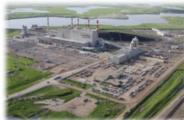
Boundary Dam, Canada is the world's first commercial scale CCS power project – post combustion coal, 115MW, opened 2014
