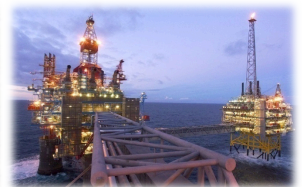
The Sleipner Project, offshore Norway, is storing 1M tonnes of CO2 per year and has been operating since 1996
