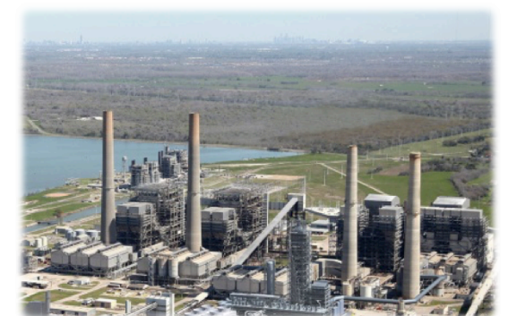
Petra Nova, US, 250MW coal is under construction and in operation in 2016
